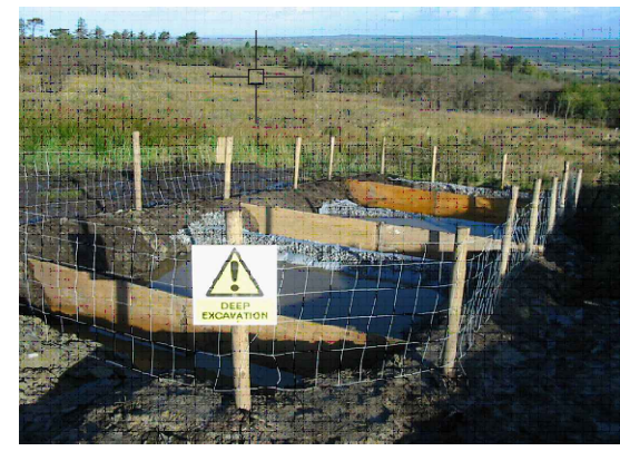
COMPLETED SETTLEMENT POND SYSTEM
